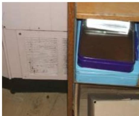
Where fan convectors are used, ensure that filters are cleaned regularly as part of routine maintenance as dirty filters will restrict airflow.
